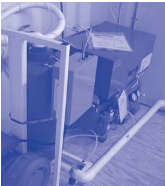
Dry vacuum pump systems eliminate water use and save energy in medical and dental applications.
