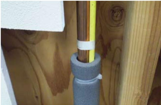
■ **Figure 4.** Photo shows self-regulating electrical heat trace strapped to the copper pipe and wrapped in insulation.
