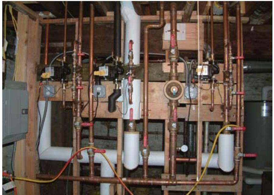
■ **Figure 2.** Photo shows three demand-controlled pumping systems, one for each wing of 12 units in a 3-story apartment building in San Francisco, CA, during major renovation. The pump for each wing is activated by a flow switch. Each unit is sub-metered for both hot and cold water and has its own demand-controlled pump activated by time-delayed motion sensors. The three main pumps each run less than 1 hour per day, and the pumps in each unit run about 15 minutes per day.
