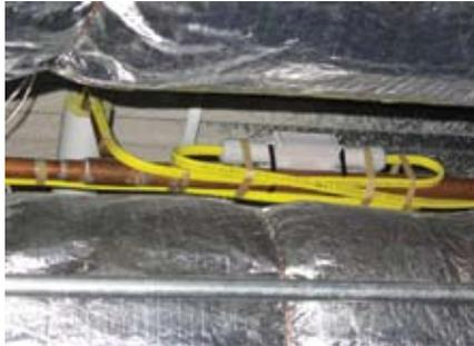
■ Photo shows a junction between two sections of self-regulating electric heat trace. The heat trace is mechanically strapped to the pipe. You can see 3/4 inch wall thickness insulation on the 3/4 inch pipe in the background. Source: Craig Drake, Tyco Thermal.
