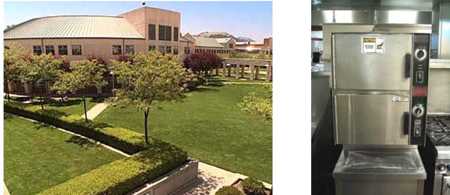
Figure 10. NC1a Corporate Cafeteria Kitchen and Boiler-based Steamer
