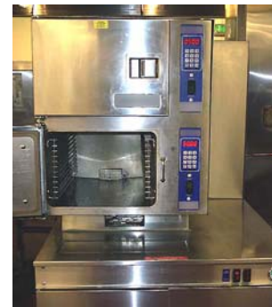
Figure 7. SC4 Hotel Banquet Kitchen and Boiler-based Steamer
