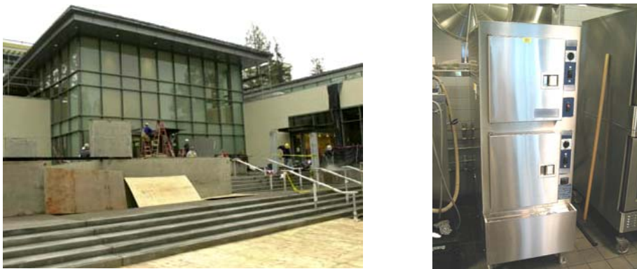
Figure 13. NC3a University Cafeteria Kitchen and Boiler-based Steamer
