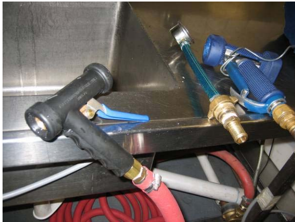
Figure 8 - New spray gun of flowrate 12L/min 'cleans much better' than old gun with flowrate 30L/min at 800kPa
